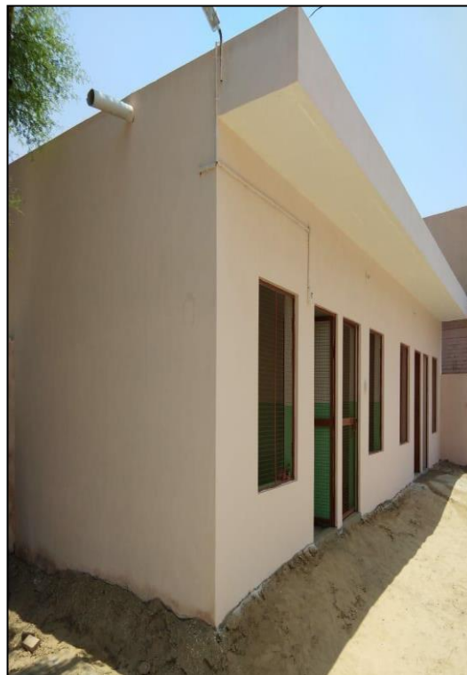
Figure 6.1:- Rescue Center in Range complex, Abohar:
